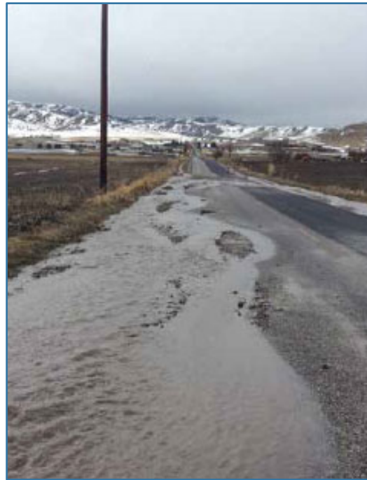
Shoulder eroded
