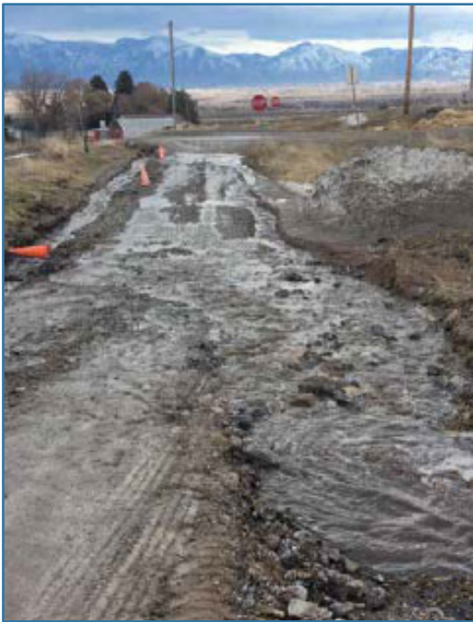
Roadway washed out
