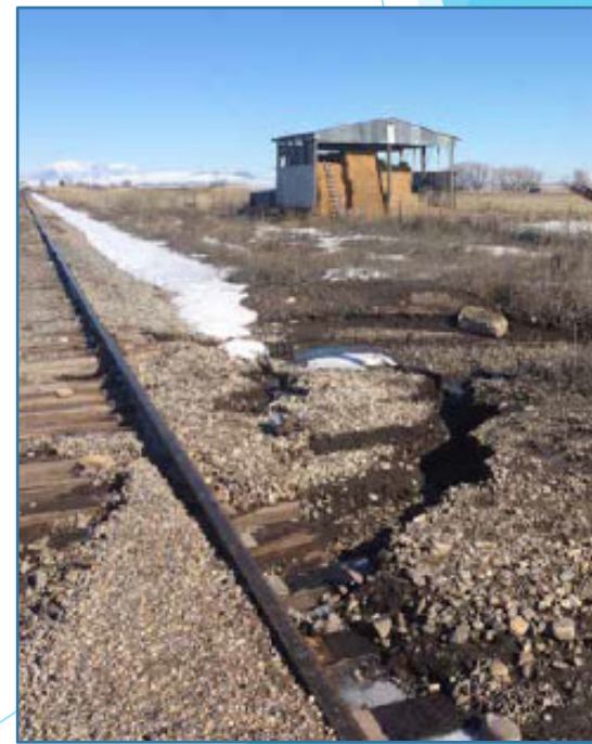
Gravel flow onto railroad tracks
