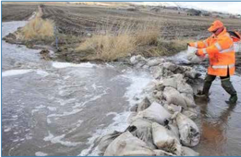
Sandbagging along SR-23 in 2012
