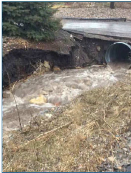
Culvert and bank erosion
