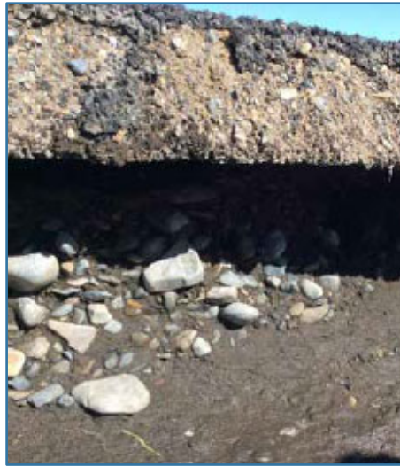
Undercut roadway, closeup
