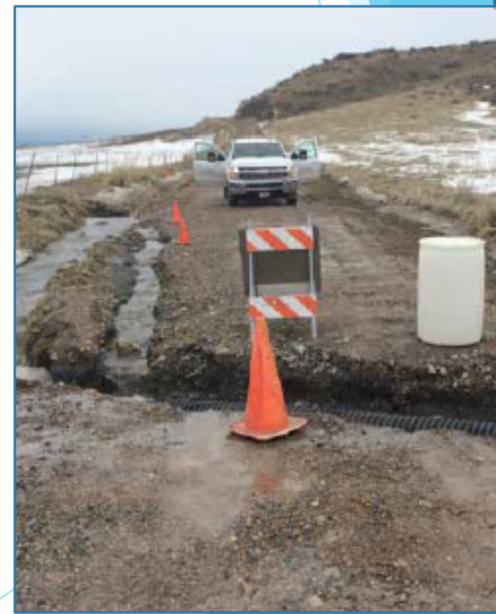
Failed Culvert
